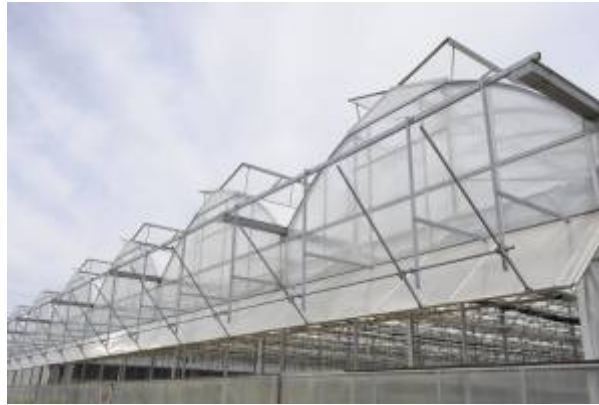
Figure 11: an example of naturally ventilated greenhouse[12]
