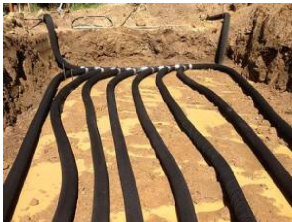
Figure 5: Air circulation tubes[4]
