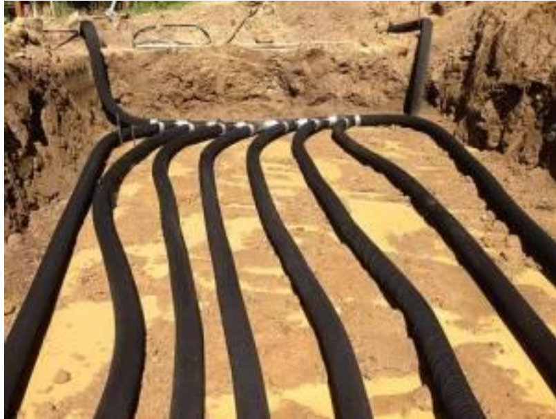
Figure 5: Air circulation tubes [4]
