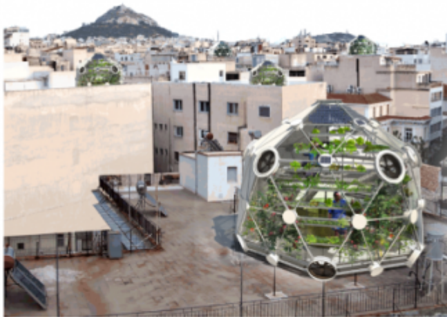
THE GLOBE (GLOBE) IS A GEODESIC GREENHOUSE STRUCTURE DESIGNED TO GROW ORGANIC FISH AND VEGETABLES USING AQUAPONIC TECHNIQUES ON AN URBAN ROOFTOP. GLOBE IS A SOLUTION THAT REDISTRIBUTES THE CONCENTRATED LOAD OF A FISH TANK OVER A LARGER SURFACE, ALLOWING THE FEASIBILITY OF AQUAPONIC FARMING IN A WIDE RANGE OF FLAT ROOFTOPS IN URBAN ENVIRONMENTS.
