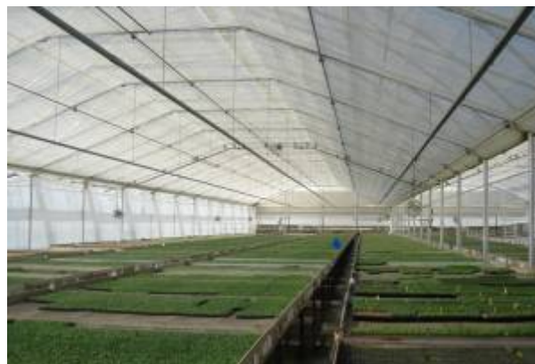
Figure 9: Thermal curtains in a big scale greenhouse [6]
